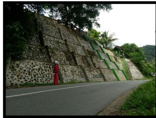
Figure 4. Building retaining walls in SDN 4 Mappatongko
