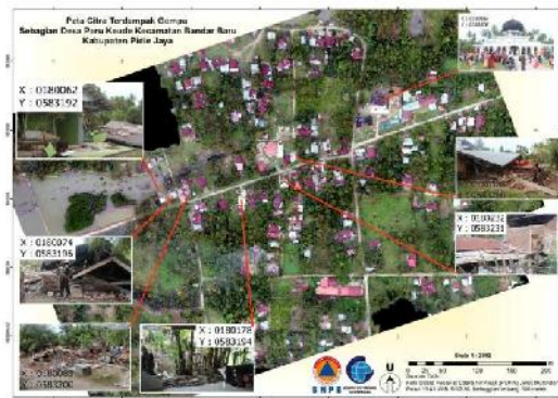
Figure 8. One of the villages affected by the 2016 Pidie Jaya Earthquake, namely Paru Keude village, Bandar Baru sub-district, Pidie Jaya district. Damage distribution of buildings has been mapped with unmanned aerial aircraft (PUNA / drone) as a result of cooperation between BIG, BNPB and a number of institutions.
