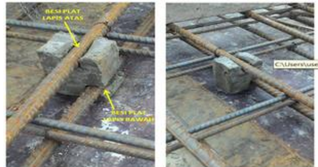
Fig. 3 Installation of modified concrete
