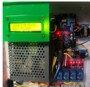
Figure 11. Water pump testing results 4
