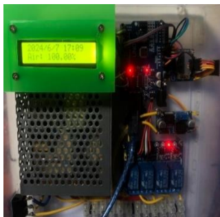
Figure 7. Waterpump 1 trial results at 08:00 to 17:00
