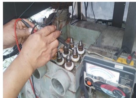
2b. Measurement of harmonic distortion
