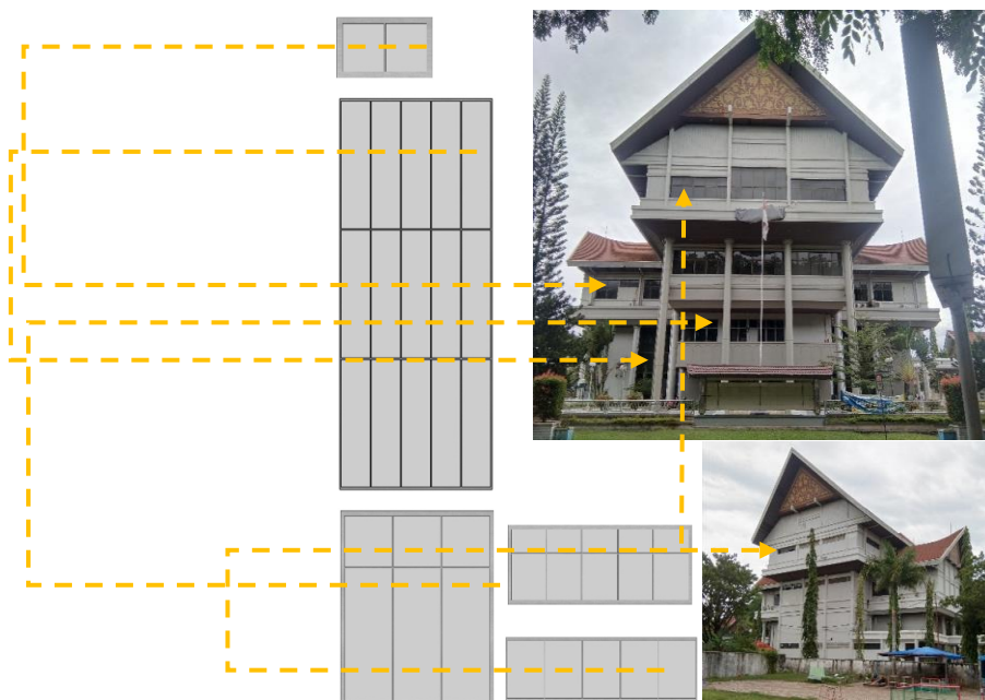
Figure 4. 6 Windows opening at the BSI bank Lhokseumawe City
