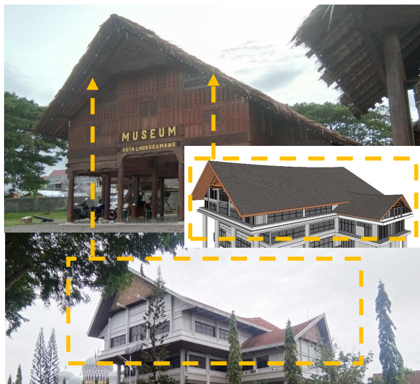
Figure 4. 11 The shape of the roof on the BSI bank in Lhokseumawe
