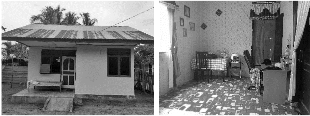
Figure 8 Exterior and interior appearance of type 2
